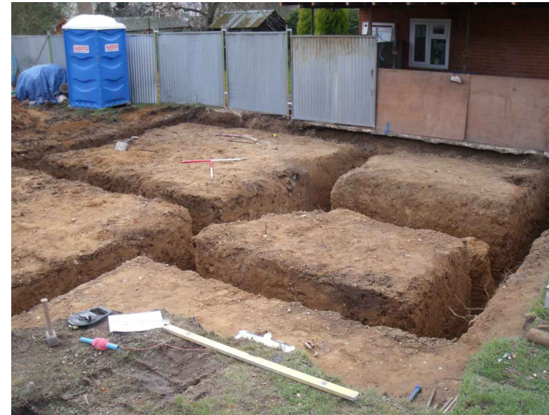
DP 5: House Foundations Post Exc - view S
