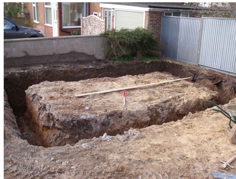
DP 7: Garage Foundation Post Exc - view S
