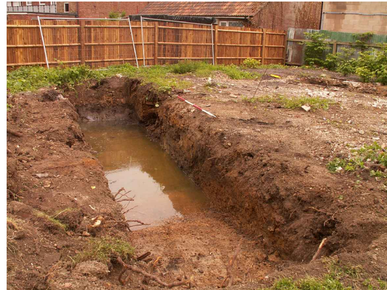
DP8 SS4, Post-excavation, Looking SW
