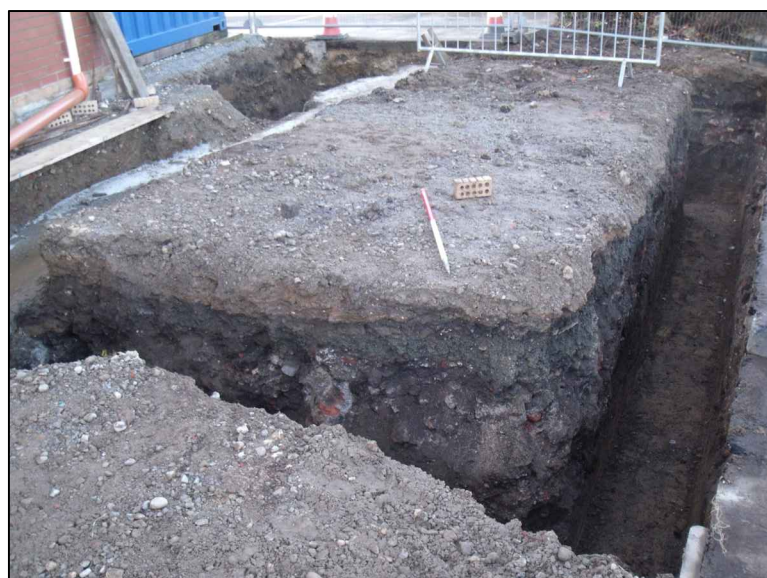
DP 3: Post Excavation - Looking W
