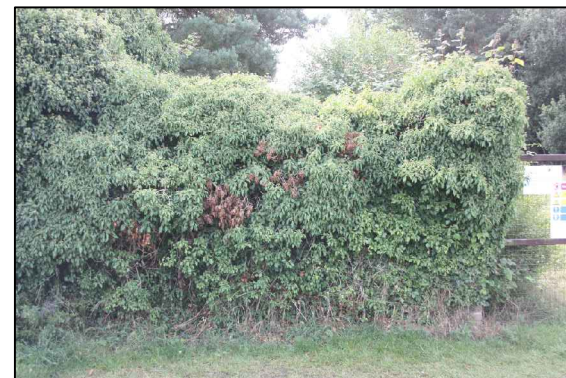
DP 10: Surviving Engine Room Building, Obscured by Plants - View S
