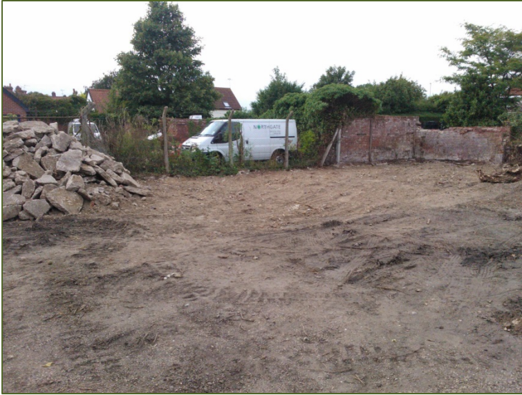
Site shot, looking north-west towards area of TT1.
