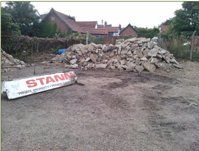
Site shot, looking west towards area of TT2.
