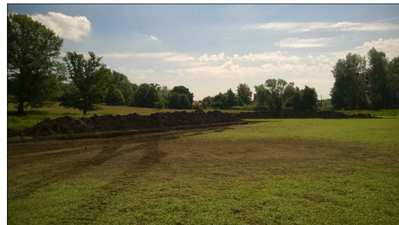
DP12: General Site Shot - View SE
