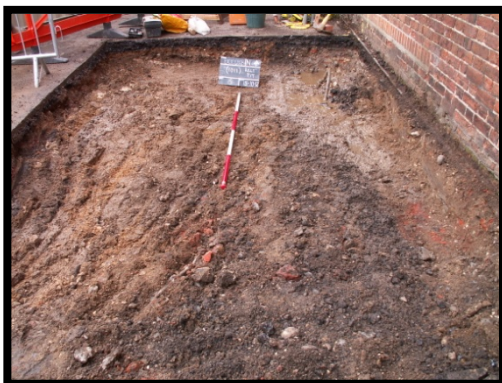
DP7: Post Excavation – Concrete Pad Area, Facing SSW.
