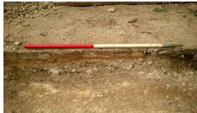
DP3; Retaining Wall Foundation, Sample Section 3, Looking N
