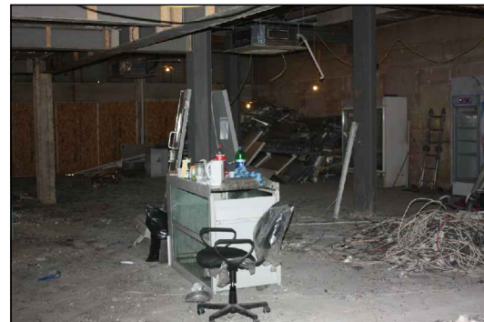
DP 2: Main Room Ground Floor - View SW
