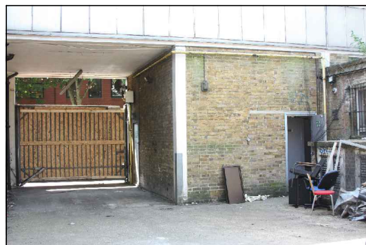
DP 4: Courtyard & Main Entrance - View SSW
