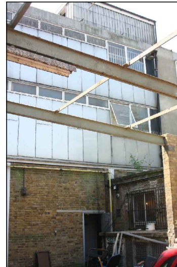
DP 3: Rear Elevation from Courtyard - View SW
