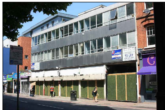
DP 7: Building Exterior Fronting On To Upper Richmond Rd - View NW
