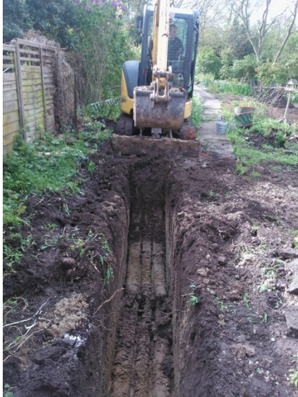
DP5: Shot of rear extension foundation trenches, facing SE.
