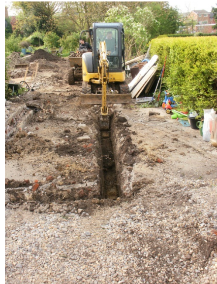
DP8: Shot of garage foundation trench excavation, facing SE.
