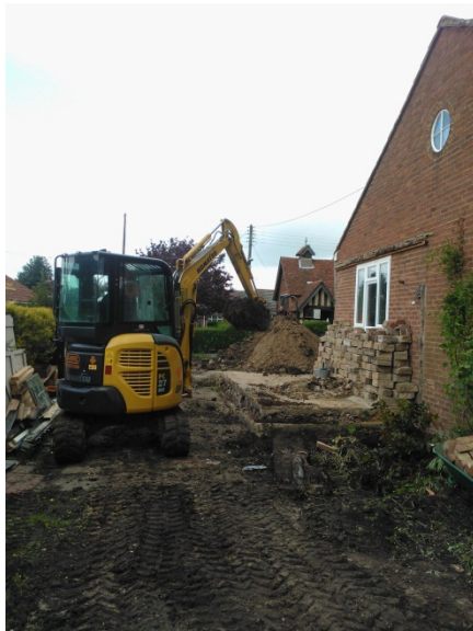
DP7: Shot of garage foundation trench excavation, facing N.
