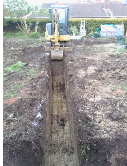
DP6: Shot of rear extension foundation trenches, facing SW.
