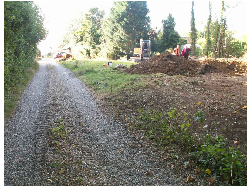
General site shot looking south
